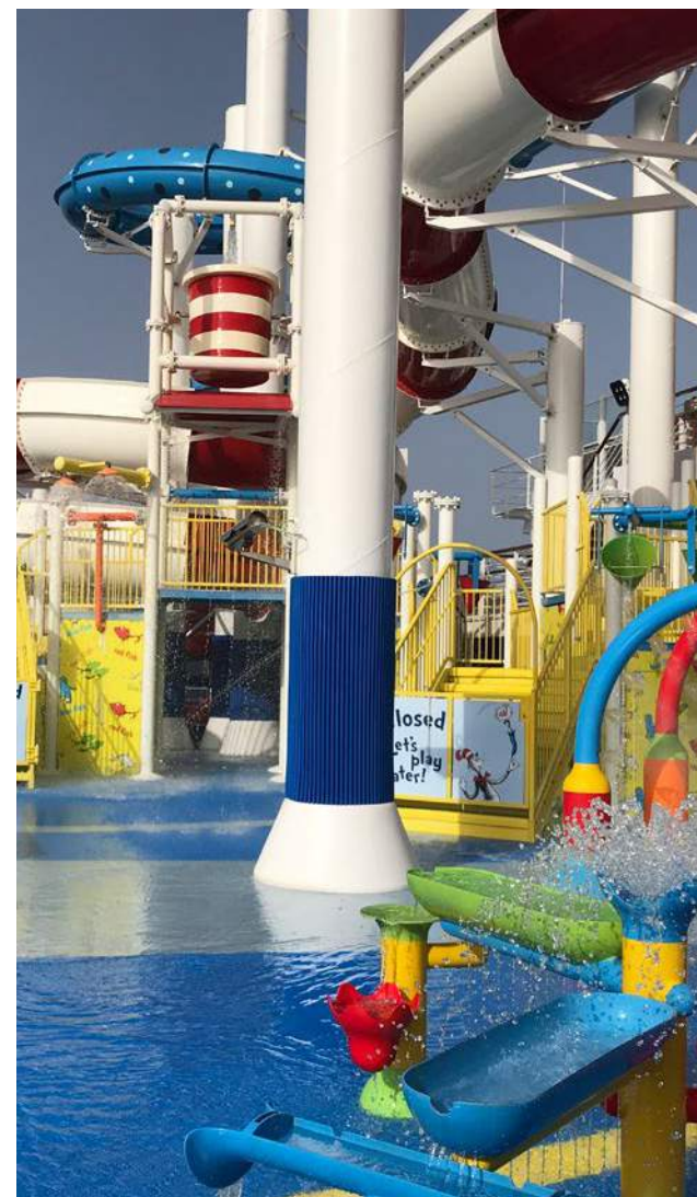
PILASTRI ACQUAPARK | MAXIONDA 28 MM
